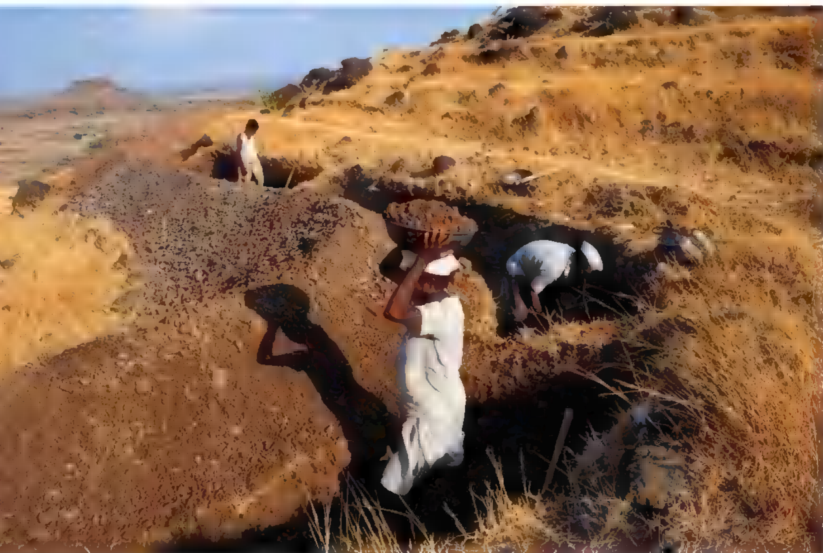
During a three-year watershed project, residents of Satichiwadi dig a trench to catch rain as it races downhill. Landless villagers are paid for this work. Landowners, whose fields will benefit from the resulting rise in the water table, donate some of their labor.
